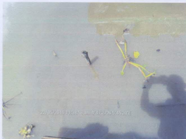
FIG A: Incident point on arrival
